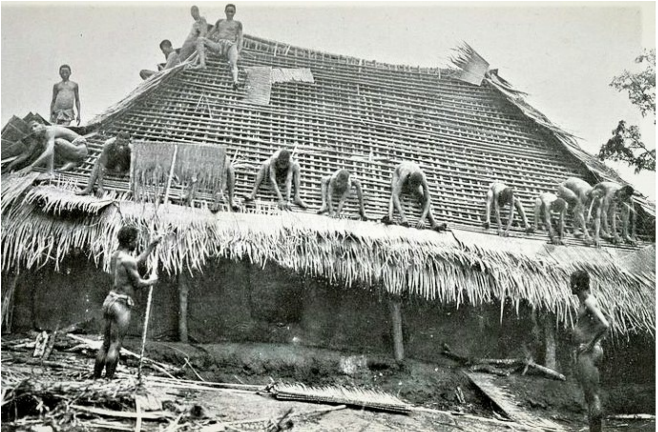
Thatching a traditional house with palm leaf mats among Igbo people of Nigeria – Author G.T. Basden, Among the Igbos of Nigeria , Wikimedia
