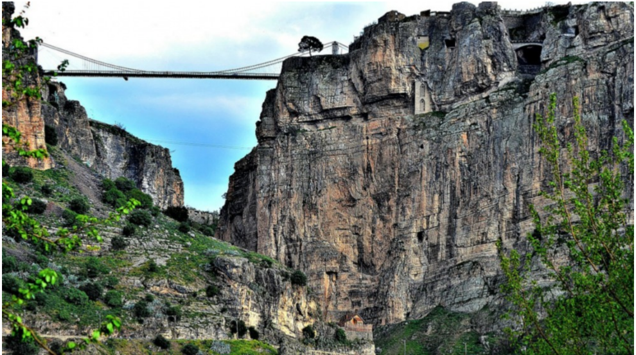
Bridge over the Gorge of Rummel, Constantine, Algeria – Author, Louadfel, Wikimedia
